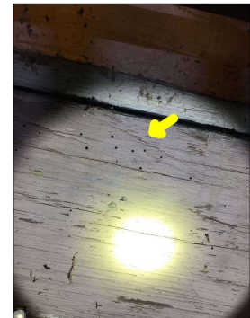
Exit holes observed. Exit holes are an indication of an infestation of powderpost beetles. Powderpost beetles are a wood destroying insect and can cause structural damage and property damage.
