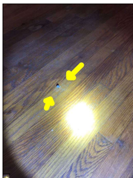
Unconventional nails sticking out from the floor.
