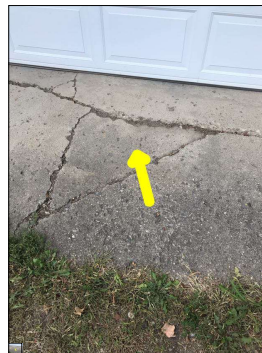
Cracks and deterioration along the driveway.
