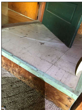
9" X 9" floor tiles. These tiles are potentially asbestos based tiles. Asbestos based products are considered a potential health/safety hazard.
