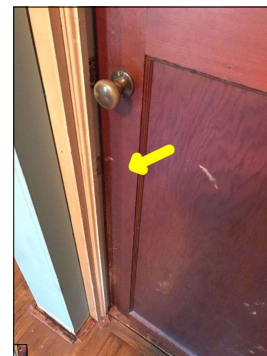
The door rubs the frame during operation.
