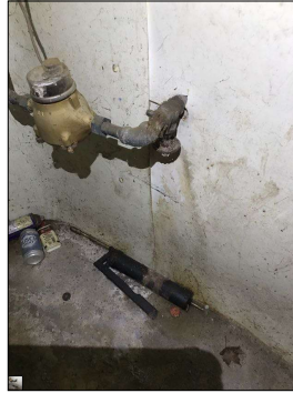
Main water shut off valve.
