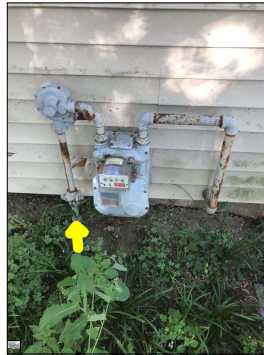
Main fuel shut off valve.
