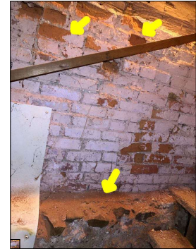
Deterioration along the foundation wall. This is considered abnormal and a defect
