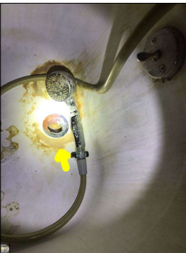
Missing drain stopper.
