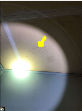
Discoloration along the ceiling tiles.
