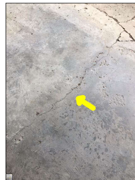
Cracks and deterioration along the floor.
