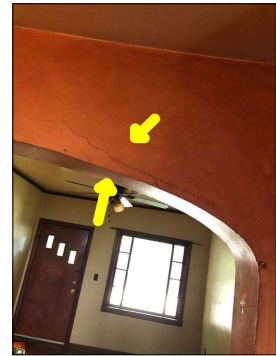
Cracks along the walls.
