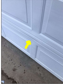
Dents/damage along the overhead garage door.
