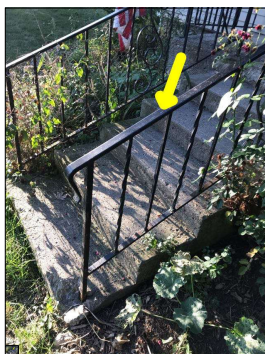
Loose handrails.
