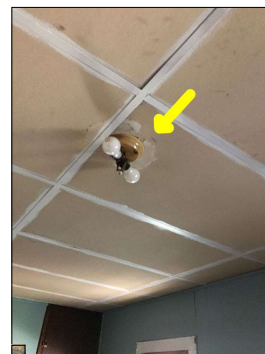
The ceiling light is missing its globe/cover.
