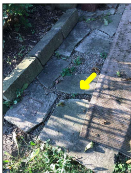
Uneven surfaces along the service walks.
