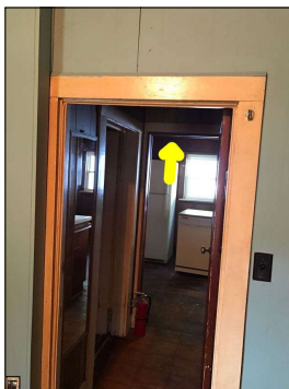
Low overhead clearance. This is a potential safety hazard.
