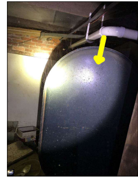
Aged oil tank observed in the basement.
