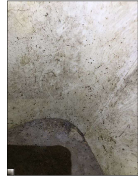
Mold like substance. An active or intermittent water source can cause mold growth and property damage.
