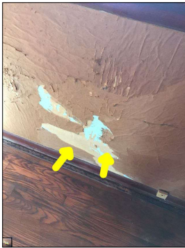
Flaking and peeling along the walls.
