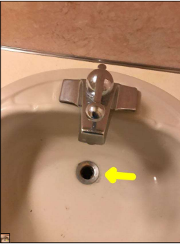
Missing drain stopper.
