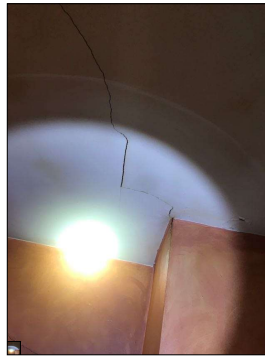
Cracks along the ceiling.
