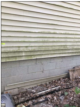
Discoloration along the siding.
