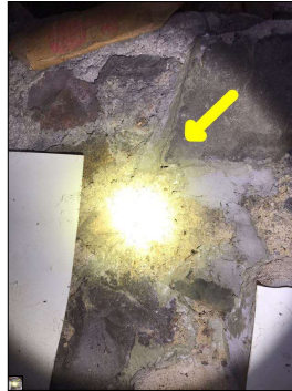
Deterioration along the field stone foundation.
