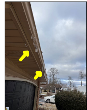
Excessive icicles hanging from the gutter system. This is considered abnormal. This could be an indication of clogged gutters, poor attic ventilation, or poor attic insulation. The excessive icicle accumulation can lead to ice dams and potential water intrusion along the eaves. Ice damming is when snow and ice prevents the roof from properly shedding water, thus allowing water to get underneath the shingles and into the house.
