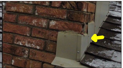
The flashing does not go up at minimum 4 inches along the base of the chimney. 4 inches is the recommended minimum height that flashing should go up around the base of the chimney. The flashing should also be cut into the chimney and sealed to prevent leakage. The current flashing along the chimney is considered subpar and amateur craftsmanship. Amateur craftsmanship is prone to failure and leakage.
