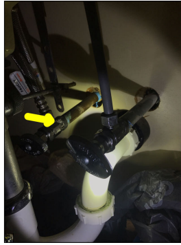
Rust/corrosion along the plumbing pipes.
