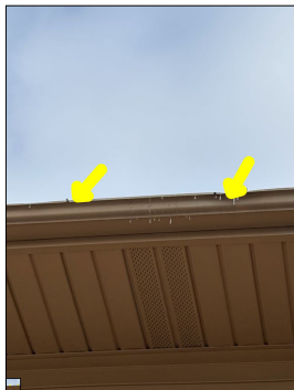
Dents/damage along the gutter system. Dents/damage along the gutter system. Also, loose gutter spikes.
