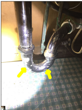
Rust/corrosion along the plumbing pipes.
