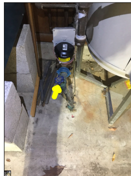
Main water shut off valve.
