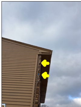
Unconventional tape and foreign substance along the siding.
