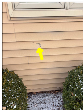
Damaged siding.
