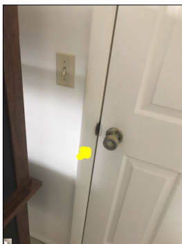
The door does not latch properly.
