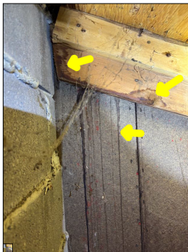
Discoloration along the sheathing/framing. Discoloration can be a potential mold like substance. An active or intermittent water source can cause mold growth and property damage. This is adjacent to the chimney/chase.
