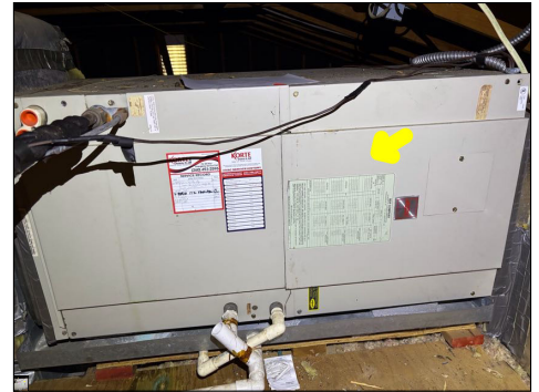
Air handler observed in the attic. This is for the central cooling.
