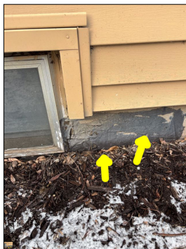
Signs of previous repairs along the foundation.
