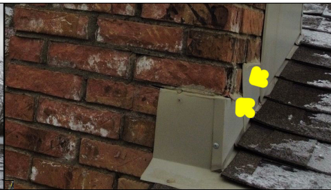
Gaps along the flashing and deterioration along the brick. These types of defects are potential leak points.
