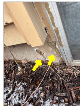
Signs of previous repairs along the foundation and a foreign substance along the foundation. Recommend a general contractor further evaluate and make necessary repairs.
