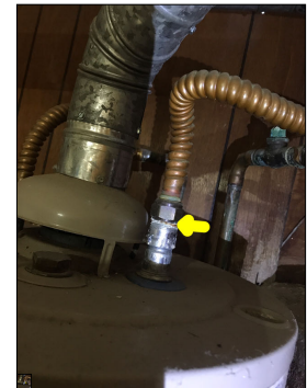
Corrosion along the water supply lines.
