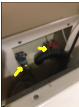
Rust/corrosion along the washer hook up lines.
