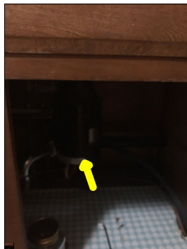
Inoperable garbage disposal. It only makes a humming noise when turned on.
