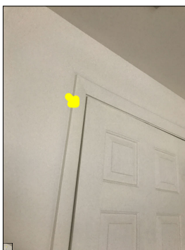
The door rubs the frame during operation.
