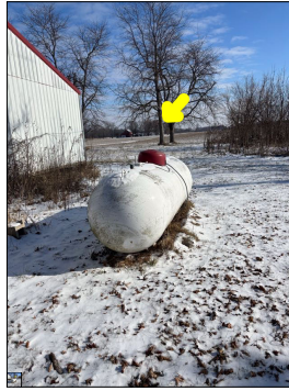
Main fuel shut off valve.
