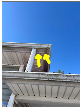
The gutter system leaks. This is considered abnormal and a defect. It appears water is getting behind the gutter as it flows from the roof. This is considered a defect.
