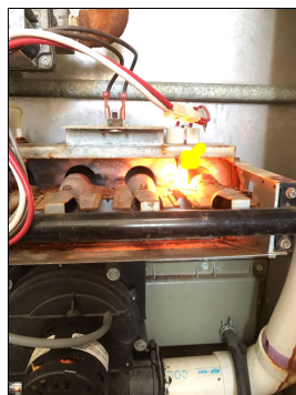
The burners never turned on, only the igniter would glow. The emergency heat/furnace is inoperable.
