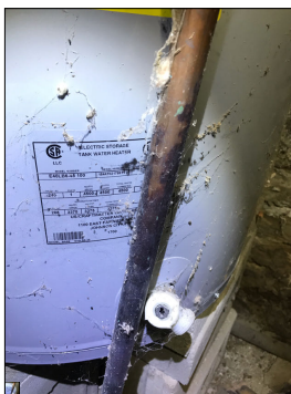
Water heater data plate.
