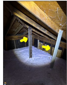
Added supports/webbing observed in the attic. This is an indication of previous structural repairs.
