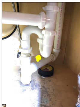
S-trap underneath the sink. S-traps no longer meet modern day plumbing standards. S-traps have the potential to siphon and become dry, thus creating the potential to allow sewer gases into the house. S-traps have the potential to make a knocking/gurgling sound when draining.
