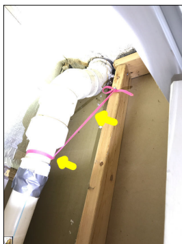
Unconventional shoe string holding the exhaust pipe up.
