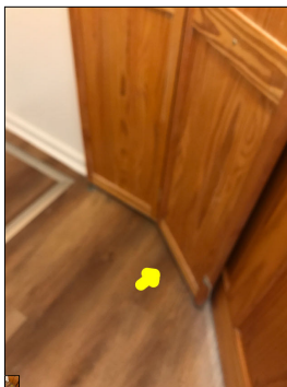
The door is detached from its track.
