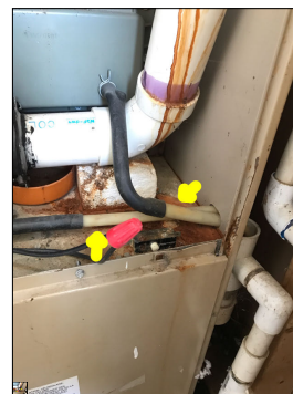
Rust and corrosion within the furnace cabinet. This is considered a defect. An active or intermittent water source can cause property damage.
