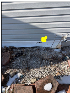
Damaged siding.
