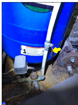
Apparent main water shut-off valve.
