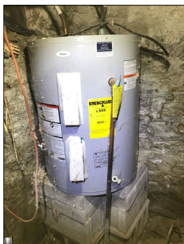
Water heater. Please note, there was no hot water on the day of the inspection.
