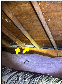
Areas of ice observed in the attic. This is an indication that the attic is not properly ventilated and/or insulated. An active or intermittent water source can cause mold growth and property damage, such as wood rot, water staining along ceilings, and damage to building materials.
