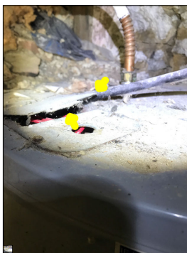
Wires routed through the knockout without a bushing or clamp. This is considered a safety hazard as the metal edge of the knockout could penetrate the wires, thus causing spark and a fire.
