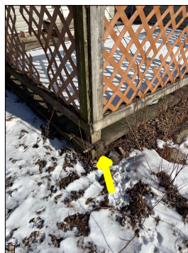
The deck has wood to soil contact. This is not a recommended practice. Water and moisture from the soil/earth can wick up along the deck and the water can be absorbed by the deck. An active or intermittent water source can cause property damage, such as wood rot damage. Also, the wood to soil contact can enable the infestation of wood destroying insects, such as termites or powderpost beetles.
