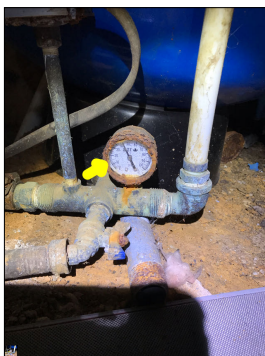
The well pressure was approximately 45 PSI during the inspection.
