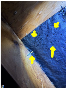
Areas of moisture observed in the attic. This is an indication that the attic is not properly ventilated and/or insulated. An active or intermittent water source can cause mold growth and property damage, such as wood rot, water staining along ceilings, and damage to building materials.
