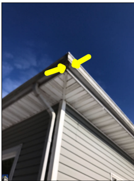
The gutter system leaks. This is considered abnormal and a defect.
