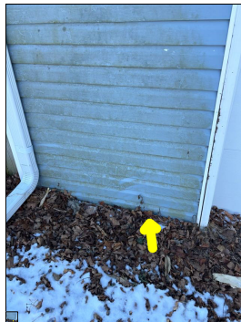
Damaged siding.
