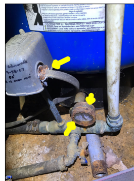
Rust/corrosion along the pressure tank components.
