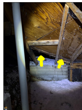
Damaged sheathing.
