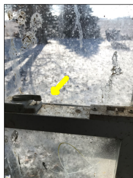
The lock does not catch the latch keeper.
