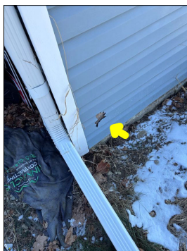
Damaged siding.
