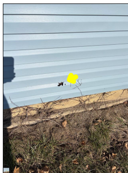
Damaged siding.
