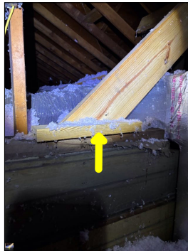
Added supports/webbing observed in the attic. This is an indication of previous structural repairs.
