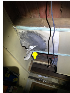
Mold like substance. An active or intermittent water source can cause mold growth and property damage.
