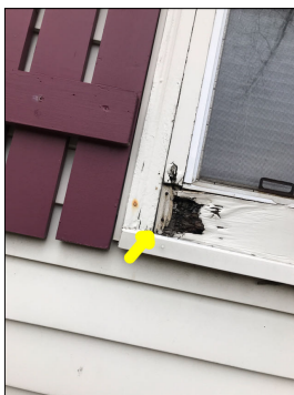
Wood rot damage.
