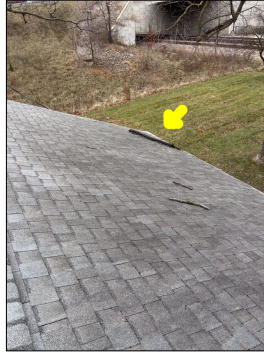
Tree branches observed along the roof. Falling tree branches can cause damage to the roof system, thus resulting in water intrusion into the attic/house.
