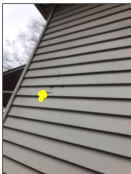
Holes along the siding.
