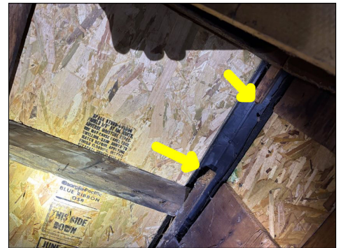
The ridge has unconventionally been cut. This is considered abnormal and a defect.
