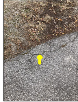
Cracks and deterioration along the driveway.
