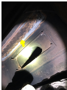
Rust and corrosion within the firebox.
