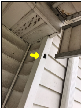
Holes along the siding.
