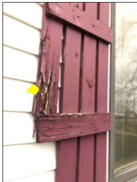
Wood rot damage along the shutters.
