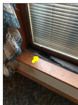
Wood rot damage along the windows.
