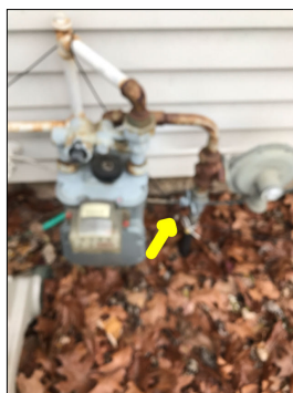
Main fuel shut off valve.
