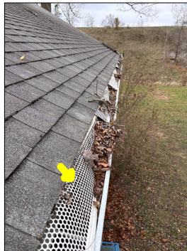
Displaced gutter guards.
