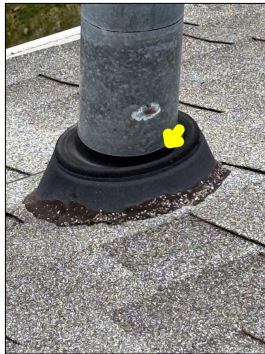
The rubber flashing is concave. This is considered a defect. The concave flashing will act as a trap for water and hold water and snow, thus creating a potential leak point. Flashing is not designed to hold water, flashing is designed to shed water.
