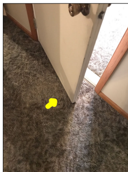
The door drags the floor during operation.
