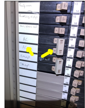
The air conditioning ( AC ) circuit breaker is oversized according to the data plate on the condenser. This is a potential safety hazard. According to the data plate, the maximum size circuit breaker should not exceed 25 amps. The current breaker is 30 amps.
