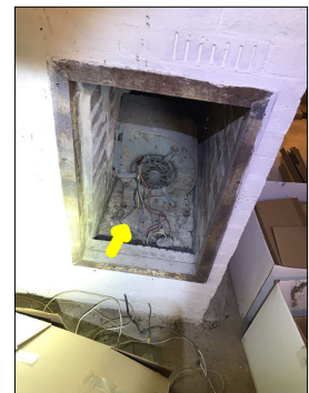
Apparent abandoned blower within the chase located in the basement.
