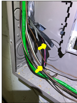
Loose/unused wires. Loose/unused wires are considered a safety hazard.
