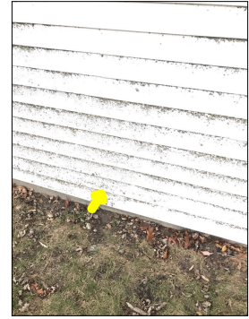
Discoloration along the siding.
