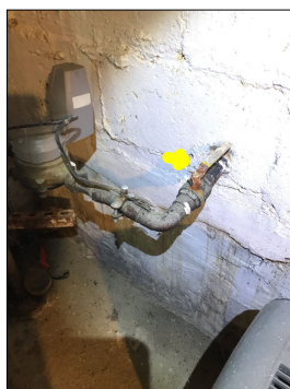
Main water shut off valve.
