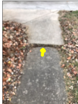
Uneven surfaces along the service walks.
