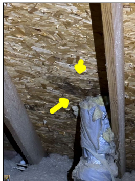
Discoloration along the sheathing. An active or intermittent water source can cause discoloration, mold growth and property damage.
