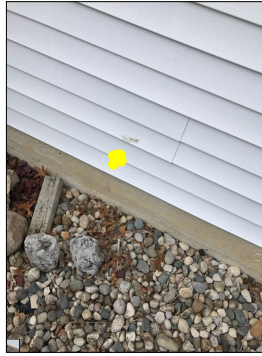
Damaged siding.
