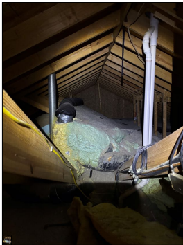
General photo of the attic.
