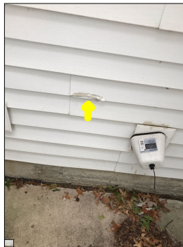
Damaged siding.
