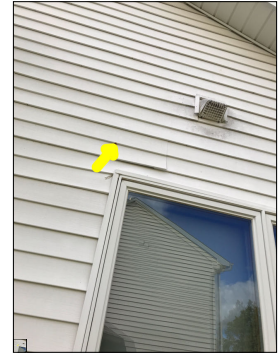
Exposed nails/fasteners along the siding. Exposed nails/fasteners are potential leak points. Exposed nails along the siding is considered amateur craftsmanship. Amateur craftsmanship is prone to failure and leakage.
