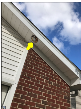
Rust and corrosion along the exterior lights.
