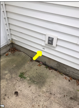
Damaged siding.
