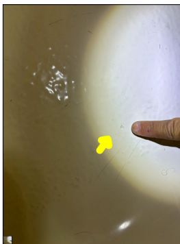
Chips along the bathtub. Chips are considered defects and are potential leak points.
