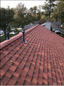
General photo of the roof.
