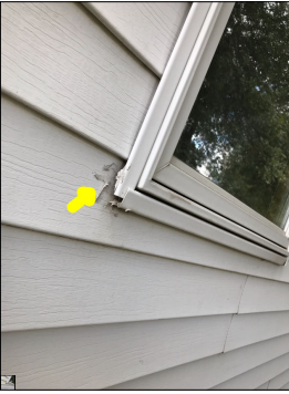
Unconventional application of caulk along the siding and unconventional repairs along the siding. This is considered abnormal and amateur craftsmanship. Amateur craftsmanship is prone to failure.
