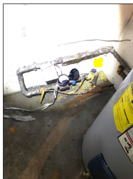
Main water shut off valve.
