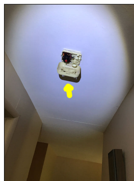
Disconnected smoke detector.
