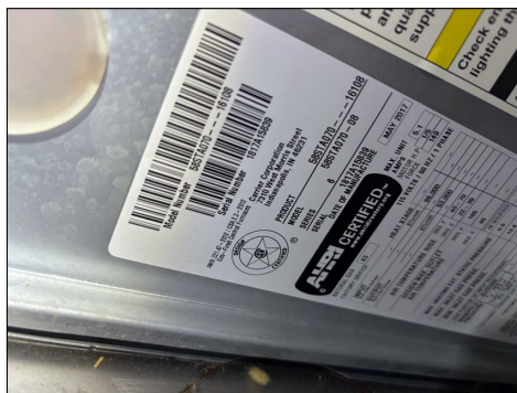
Furnace data plate.
