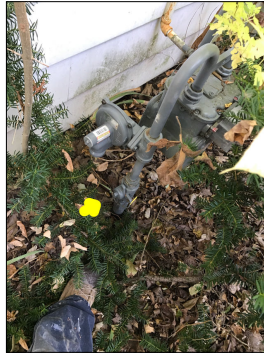
Main fuel shut off valve.
