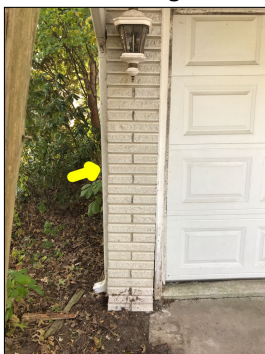
The brick siding is not plumb. It's leaning.
