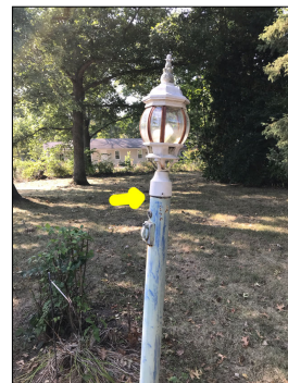
The front light post is not plumb.
