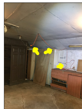
Extension cord observed. Extension cords should not be used as permanent wiring. Extension cords used as permanent wiring is considered a potential safety hazard.
