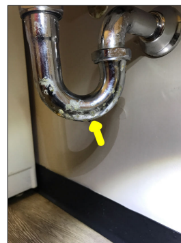
Rust/corrosion along the plumbing pipes.
