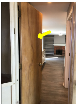
The door that separates the interior of the house appears to be a hollow door. Hollow doors are not a proper fire rated door. This is a potential safety hazard.
