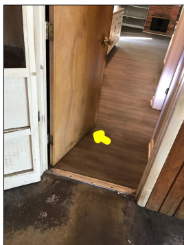
The door drags the floor during operation.
