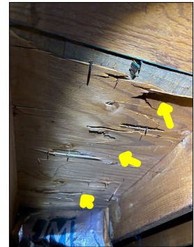
Areas of delaminated sheathing. This is considered abnormal and a defect. Delaminated sheathing is primarily caused by an active or intermittent water source. An active or intermittent water source can cause mold growth and property damage.
