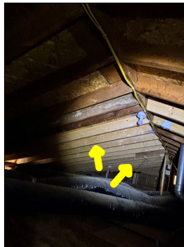
Added rafters and new rafters observed within the attic. This is an indication that the house has experienced structural repairs.
