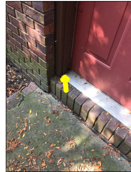
Wood rot damage along the service door.
