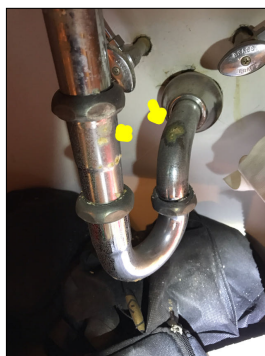
Rust/corrosion along the plumbing pipes.
