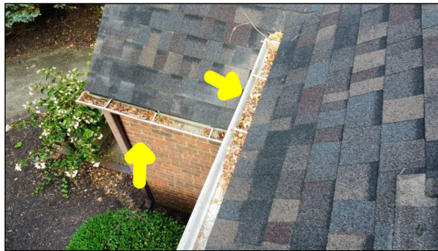
The gutter system is dirty and needs to be cleaned. A dirty gutter system can cause excessive water to accumulate around the house, thus potentially causing water intrusion into the house or potential foundation problems due to excessive hydrostatic pressure. Also, a dirty gutter system can cause excessive water to flow along the siding which could allow water to get behind the siding. An active or intermittent water intrusion source can cause mold growth and property damage.
