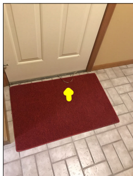
Torn weatherstrip along the door.
