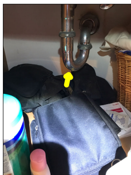
Rust/corrosion along the plumbing pipes.
