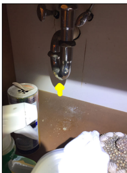
Rust/corrosion along the plumbing pipes.
