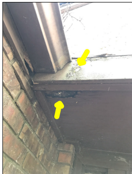
Wood rot damage.
