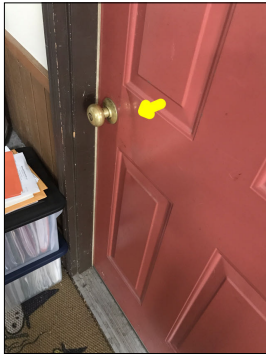
Damage/dents along the door.
