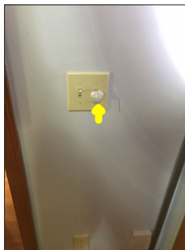
Unconventional tape along the switch. This is considered abnormal and amateur craftsmanship.
