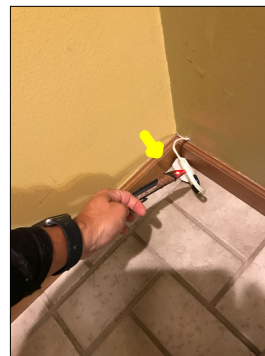
Exposed wires/unconventional wires sticking out from the wall. This is a potential safety hazard.
