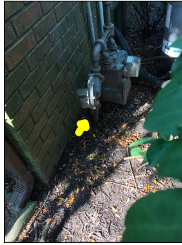
Main fuel shut off valve.
