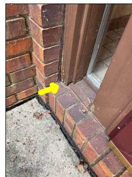
Wood rot damage.
