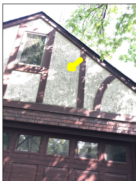
The house has stucco siding in some areas. Please note, stucco siding is prone to absorbing moisture. An active or intermittent water source can cause mold and property damage.
