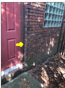
Unconventional application of caulk along the brick. This is considered abnormal and amateur craftsmanship.
