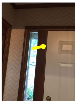
The door rubs the frame during operation.
