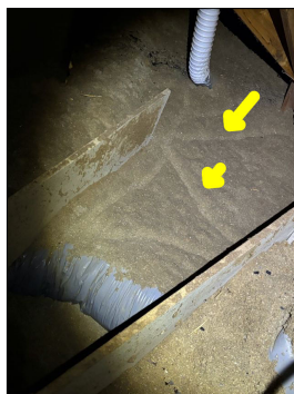
Mice/rodent tracks along the insulation. Wildlife activity can cause property damage.
