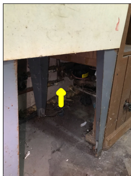
Apparent main water shut-off valve.
