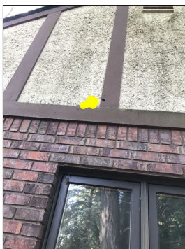
Holes along the siding.
