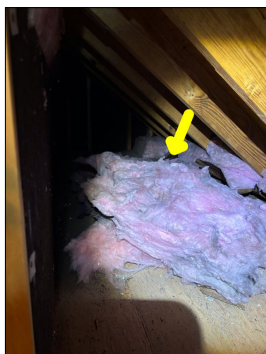
Displaced insulation. Displaced insulation is considered abnormal and a defect.
