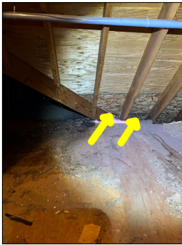
Areas of replaced sheathing. This is an indication that the original sheathing was defective. Normally, due to an intermittent or active water source.
