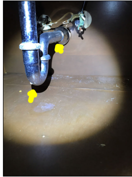
Rust/corrosion along the plumbing pipes.
