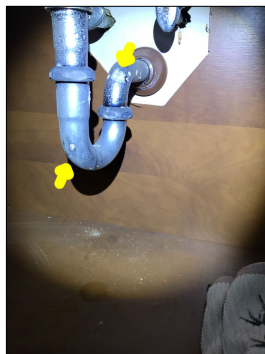
Rust/corrosion along the plumbing pipes.
