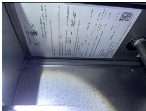
Furnace data plate.
