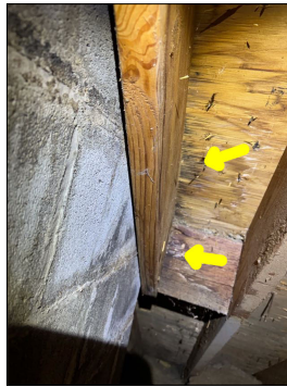
Discoloration along the sheathing. An active or intermittent water source can cause discoloration, mold growth and property damage. This is adjacent to the chimney. No moisture detected in this area on the day of the inspection.
