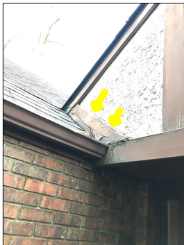
Unconventional application of caulk along the siding. This is considered abnormal and amateur craftsmanship.
