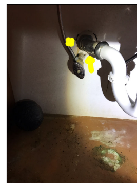
Rust/corrosion along the plumbing pipes.
