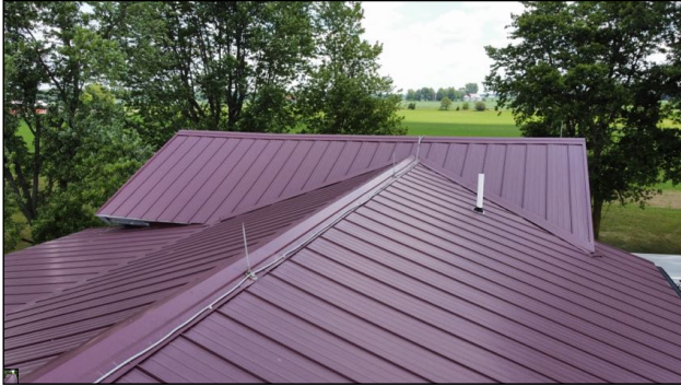
General photo of the roof.
