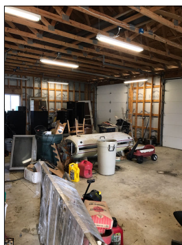
General photo of the interior of the pole barn.
