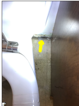
Discoloration along the wall and signs of previous water damage. An active or intermittent water source can cause mold growth and property damage.
