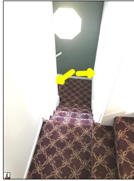
Missing handrail.
