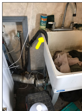
The washing machine unconventionally discharges into the sink. This is not a recommended practice and does not meet the industry standard. The washing machine should discharge into the main drain pipes. Recommend licensed plumber further evaluate and make necessary repairs.
