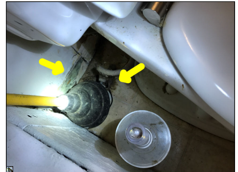
Discoloration along the wall and signs of previous water damage. An active or intermittent water source can cause mold growth and property damage.
