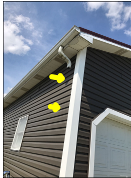
Missing downspout.
