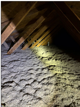
General photo of the attic.
