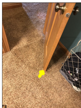
The door drags the floor during operation.
