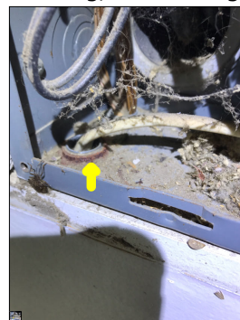
Rust and corrosion within the circuit breaker panel. This is considered abnormal and a potential safety hazard. An active or intermittent water source can cause rust and corrosion.
