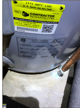
Water heater data plate.
