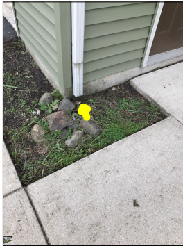
Missing downspout elbows.
