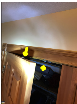
Defective door latch.
