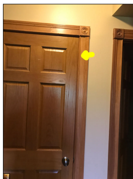
The door rubs the frame during operation.
