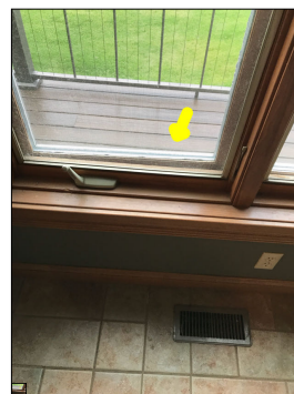
The window crank is defective. The crank is unable to close the window.
