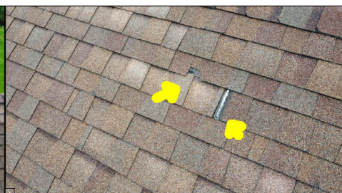
Damaged roof shingles.
