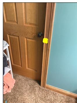
The door does not latch properly.
