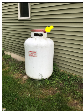
Main fuel shut off valve.
