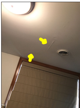
Discoloration along the ceiling and some peeling.
