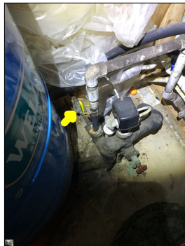
Apparent main water shut-off valve.
