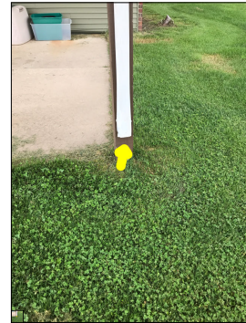
Missing downspout elbows.
