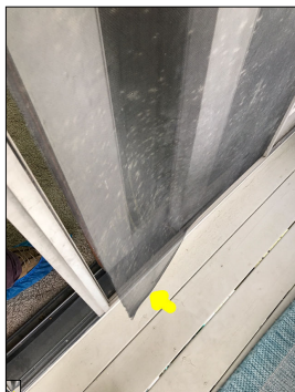
Torn screen along the door.
