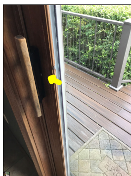
Missing knob to the lock.
