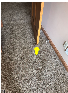
The door drags the floor during operation.
