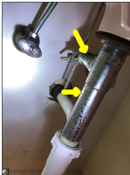
Rust/corrosion along the plumbing pipes.
