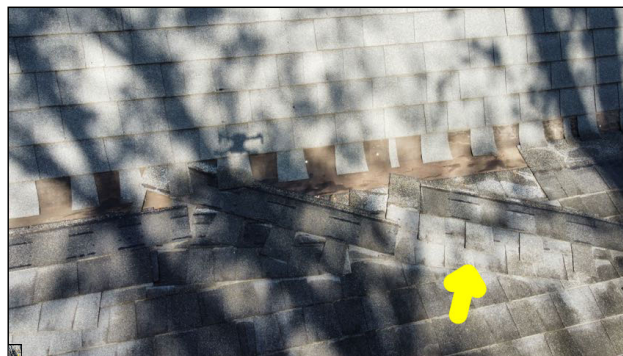
Missing/loose roof shingles.
