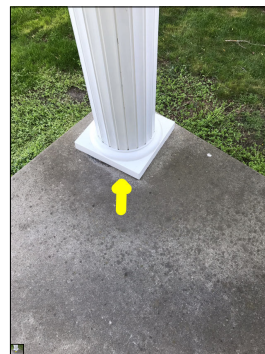
The column base is crooked compared to the other columns.
