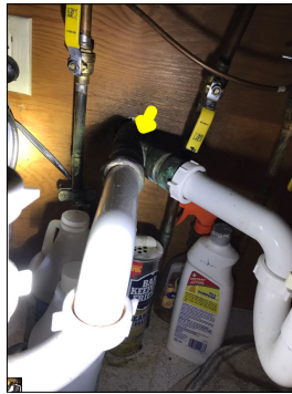
Aged copper drain pipes. Copper pipes make good water supply lines, however, they are not as effective for drain pipes. This is because copper drain pipes are thin walled, which means they are not very robust. Also, some cleaning products and house hold products are acidic which causes copper pipes to corrode. Also, urine is acidic, which can also cause copper pipes to corrode. Due to the age of copper drain pipes, repairs should be anticipated and possible replacement of copper drain pipes should be anticipated.
