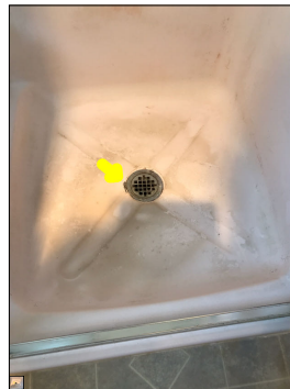
Chips along the shower. Chips are considered defects and are potential leak points.
