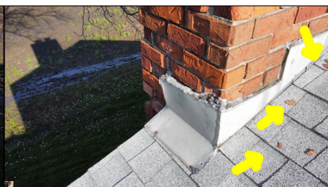
Pieces of brick from the chimney that is laying along the roof shingles. This is an indication that the chimney is deteriorating.
