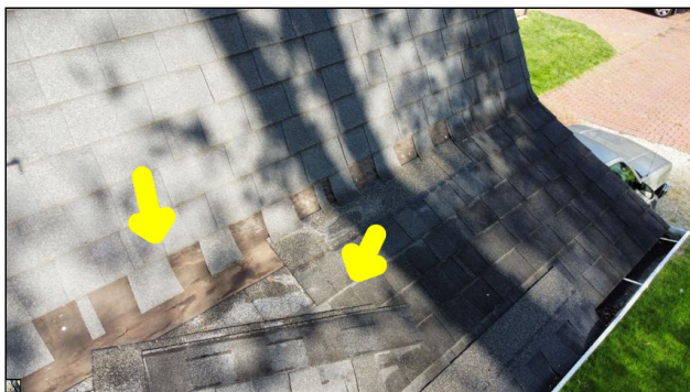
Missing/loose roof shingles.
