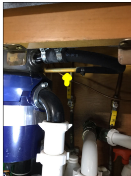
The dishwasher drain line does not have a high loop. A high loop prevents drain water from flowing into the dishwasher and contaminating the clean dishes.
