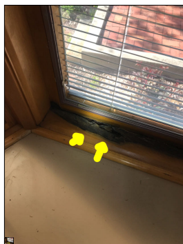
Wood rot damage along the window.
