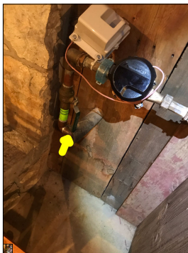
Main water shut off valve.
