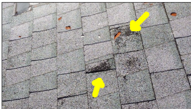
Granule loss along the roof shingles
