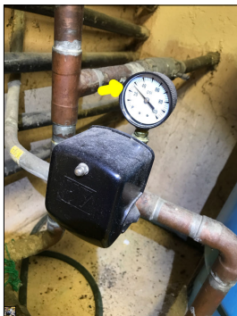
The well pressure was approximately 28 PSI during the inspection.
