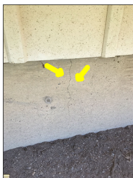
Cracks along the foundation. Cracks are considered a defect. Cracks should be repaired/sealed to prevent the intrusion of moisture, insects, wood destroying insects, mice, and radon.
