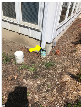
The downspout is off center from the drain tile.
