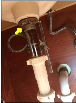
Rust/corrosion along the plumbing pipes.
