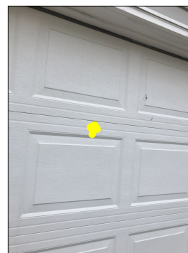
Dents/damage along the overhead garage door.
