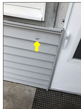
Damaged siding.
