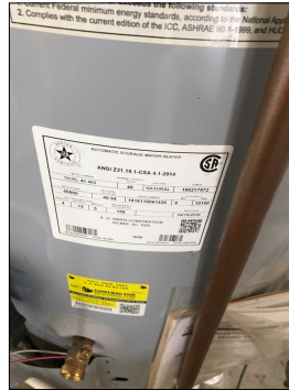
Water heater data plate.
