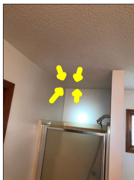
Discoloration along the ceiling.
