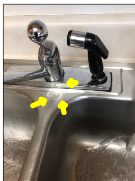
The faucet leaks during operation. A leaking faucet has the potential to leak underneath the sink. An active or intermittent water source can cause property damage and mold growth.
