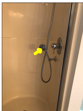
The faucet/showerhead leaks when turned off. This is considered abnormal and a defect.
