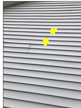
Damaged siding.
