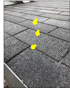
Pitting along the roof shingles.
