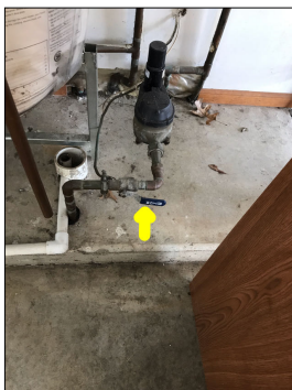
Main water shut off valve.
