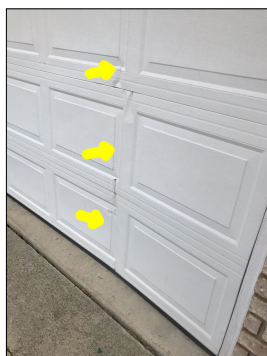
Dents/damage along the overhead garage door.
