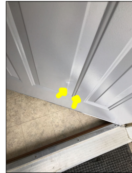
Damage/dents along the door.
