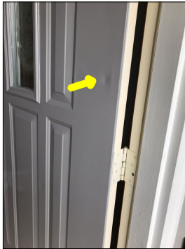
Damage/dents along the door.
