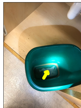
There is a bucket with water underneath the sink. This is an indication of a defective plumbing line. An active or intermittent water source can cause mold and property damage.
