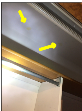
Discoloration along the ceiling.
