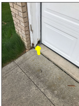
Wood rot damage.
