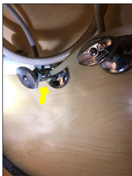
Rust/corrosion along the plumbing pipes.
