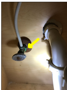
Rust/corrosion along the plumbing pipes.
