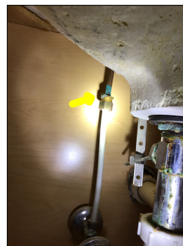
Rust/corrosion along the plumbing pipes.
