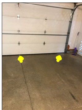
Daylight can be seen from the interior. This is an entry point for moisture, insects, mice, rodents, etc.
