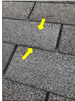
Granule loss along the roof shingles
