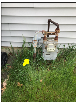
Main fuel shut off valve.
