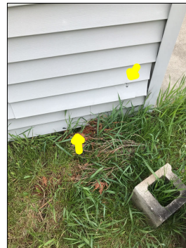
Damaged siding.
