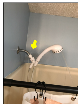
The showerhead leaks during operation.
