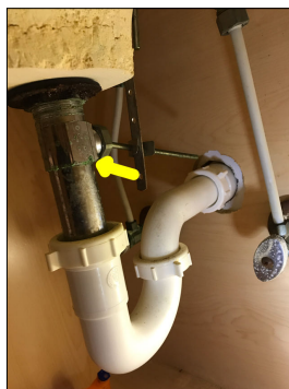
Rust/corrosion along the plumbing pipes.
