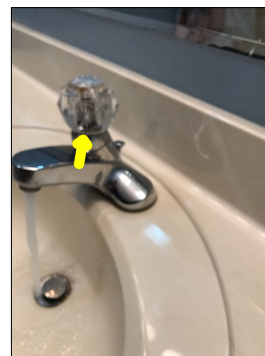
The faucet slightly leaks during operation. A leaking faucet has the potential to leak underneath the sink. An active or intermittent water source can cause property damage and mold growth.
