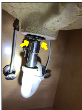
Rust/corrosion along the plumbing pipes.
