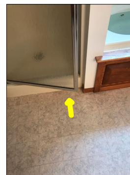
The door does not properly close.
