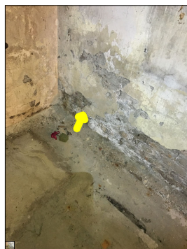
Deterioration along the foundation wall. This is considered abnormal and a defect
