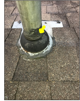
Unconventional application of roof sealant along the rubber flashing. Rubber flashing is designed to be caulkless. This is considered amateur craftsmanship. Most roof sealants are petroleum based. A petroleum based product can cause the rubber flashing to prematurely deteriorate, thus creating a leak point.
