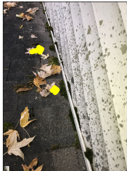
Biological growth along the roof. This is considered a defect. Biological growth has the potential to hold water. Shingles are not designed to hold water, shingles are designed to shed water.
