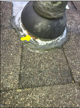
Rust and corrosion along the flashing. Rust and corrosion can create holes in the flashing, thus creating potential leak points.
