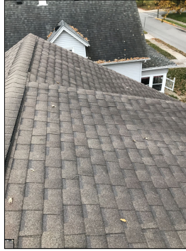
General photo of the roof.
