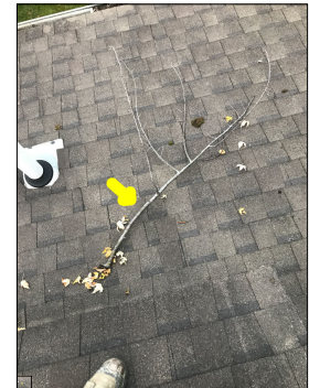
Tree branches observed along the roof. Falling tree branches can cause damage to the roof system, thus resulting in water intrusion into the attic/house.
