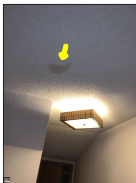
Discoloration along the ceiling. Discoloration along the ceiling is considered abnormal and a defect. An active or intermittent water source can cause discoloration, mold growth and property damage.
