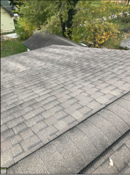
General photo of the roof.
