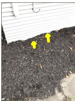
The siding is in proximity to the ground. Siding should have at least 6 to 8 inches of clearance above the ground. Maintaining proper clearances reduces access to wood structures behind the siding and helps preserve the house. The proper clearances help restrict access from wood destroying insects and/or moisture/water that might find its way behind the siding.
