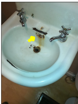
Rust and corrosion along the sink.
