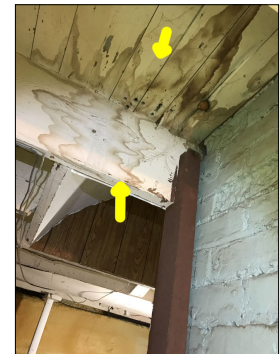
Signs of previous water intrusion and water damage. An active or intermittent water source can cause mold growth and property damage.
