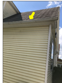
Dents/damage along the gutter system.
