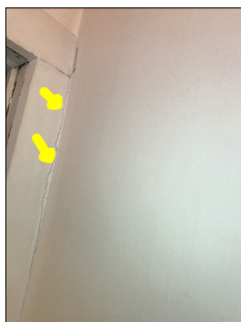
Cracks along the walls.
