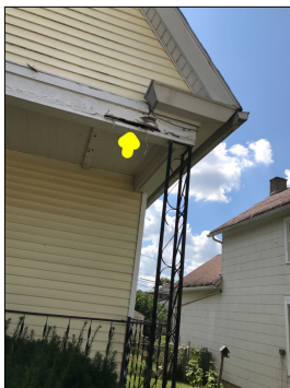
Wood rot damage.
