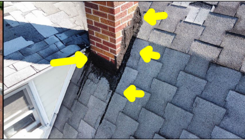
Unconventional and excessive application of roof sealant along the base of the chimney. This is considered abnormal and amateur craftsmanship. Amateur craftsmanship is prone to failure and leakage.
