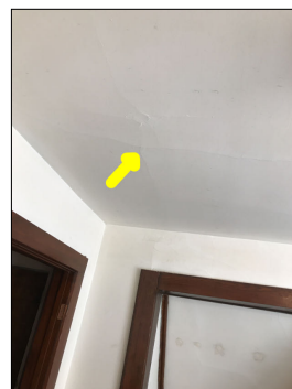
Cracks along the ceiling.
