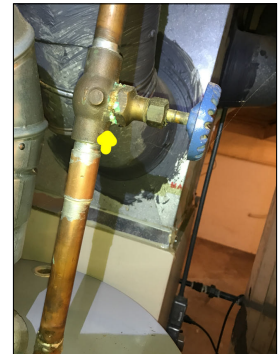
Corrosion along the water supply lines.
