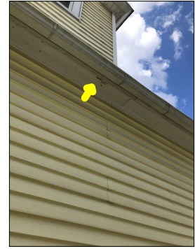
Damaged siding.
