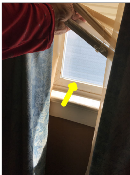
The window sash falls down upon opening the window.
