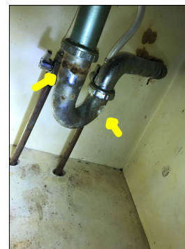
Rust/corrosion along the plumbing pipes.
