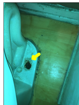
Rust and corrosion along the toilet anchor bolts. This is considered a defect and the rust and corrosion can cause the toilet to become loose and potentially leak.
