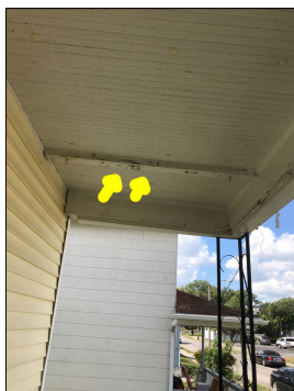
Flaking and peeling along the siding.
