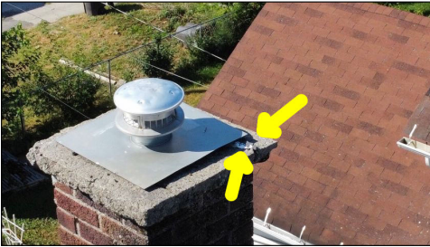
Cracks along the chimney. Cracks are considered defects and potential leak points.
