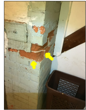
Deterioration and cracking along the chase.
