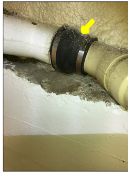
Rubber coupler observed. This is an indication that previous repairs were conducted along the plumbing lines.
