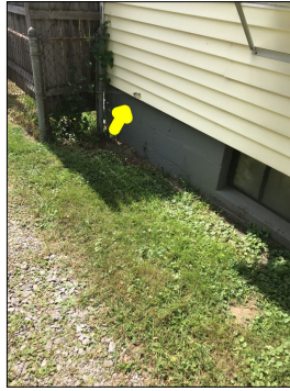
Damaged siding.
