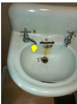
The faucet leaks when turned off. This is considered abnormal and a defect.
