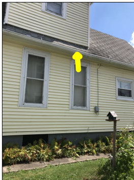
Unconventional sags along the gutter system. This is considered a defect as the sags will act as a catch for water.
