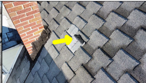
Damaged roof shingles.
