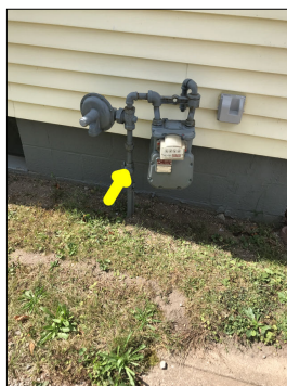
Main fuel shut off valve.
