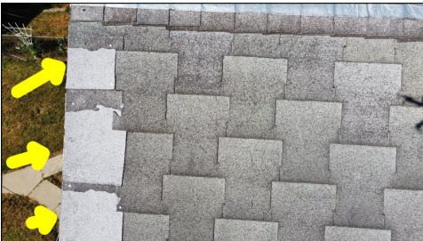
Repairs observed along the roof. The repairs are considered amateur craftsmanship. Amateur craftsmanship is prone to failure and leakage.
