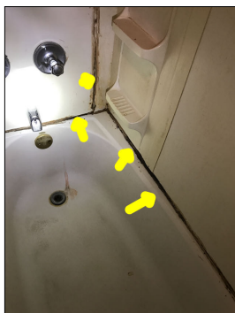
Discoloration along the bathtub. Discoloration can potentially be a mold like substance.
