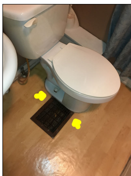
The toilet is unconventionally on top of the vent cover. This is considered abnormal.
