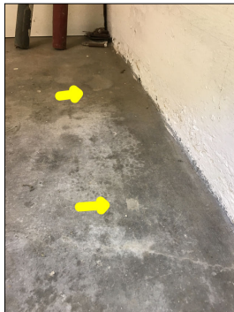
Drilled holes observed along the slab. This is an indication of previous termite treatment. Termites are a wood destroying insect and can cause structural damage to a house.
