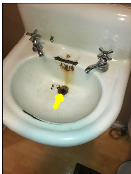
Missing drain stopper.
