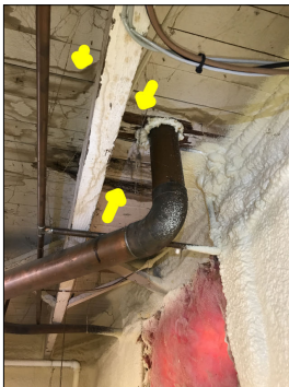
Signs of previous water intrusion and water damage. An active or intermittent water source can cause mold growth and property damage.
