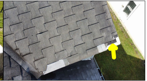
Damaged roof shingles.
