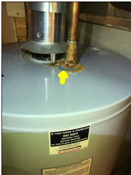
Corrosion along the water supply lines.
