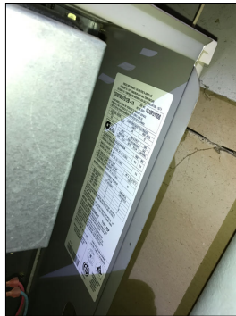
Furnace data plate.
