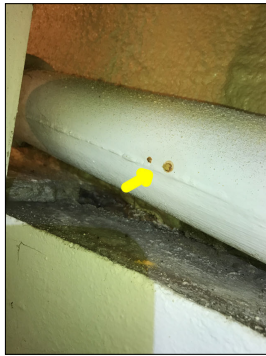
Rust and corrosion along the plumbing pipes.
