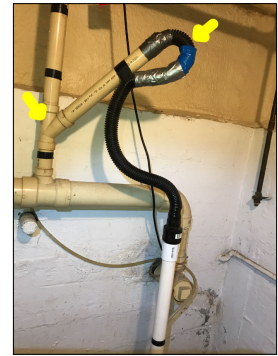
The sump pump discharges into the main drain pipes. This is not a recommended practice and does not meet the industry standard. Sump pumps should discharge to the exterior.
