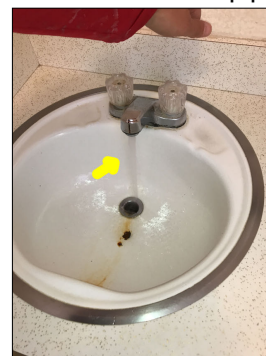
Abnormal water pressure/flow from the faucet. The abnormal water pressure/flow is causing water to splash outside the sink. An active or intermittent water source can cause property damage.
