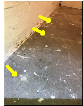
Drilled holes observed along the slab. This is an indication of previous termite treatment. Termites are a wood destroying insect and can cause structural damage to a house.
