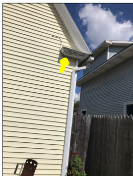
Flaking and peeling along the siding.
