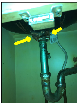
Rust/corrosion along the bottom of the sink.
