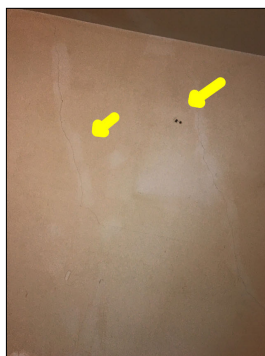
Cracks along the walls.
