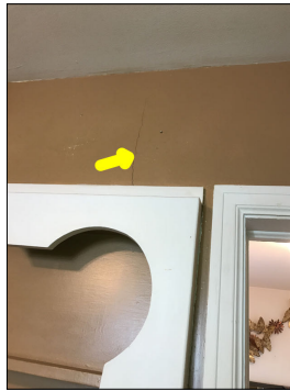
Cracks along the walls.
