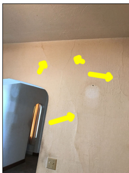
Cracks along the walls.
