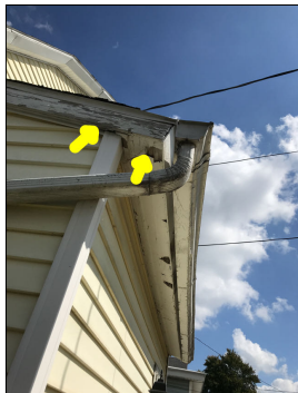
Flaking and peeling along the siding.
