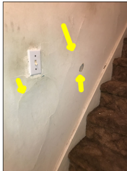
Cracks and damage along the walls in the stairwell.
