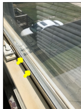
Cracks along the seal, this is a sign that the window is aged.
