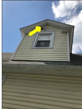
The vent cover is missing a critter guard.
