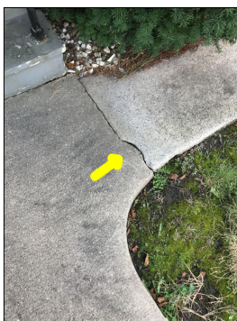
Cracks and deterioration along the service walks.
