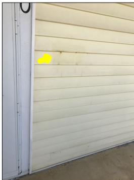
Holes along the siding.
