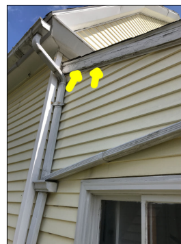
Flaking and peeling along the siding.
