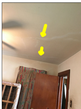
Cracks along the ceiling.
