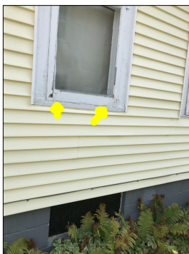
Flaking and peeling along the siding.
