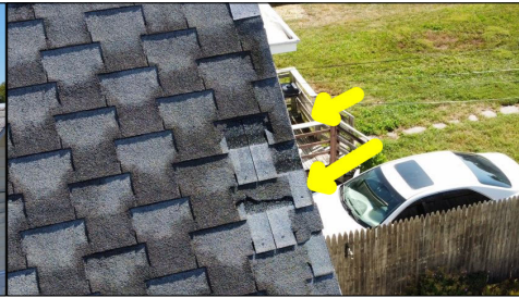
Damaged roof shingles.
