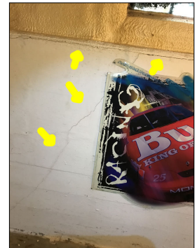
Cracks and signs of movement along the foundation walls.
