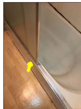
The door does not stay open. It slides to a closed position. Both shower doors have the same defect.
