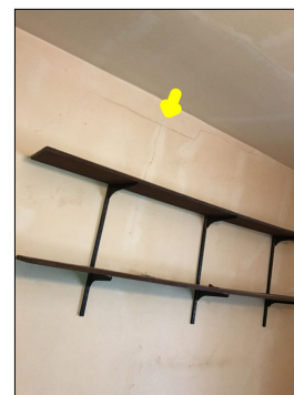
Cracks along the walls.
