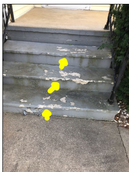
Cracks and deterioration along the service walks/steps.
