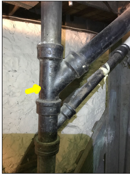
Aged cast iron drain pipes. Cast iron drain pipes no longer meet modern day plumbing standards. Cast iron pipes are prone to corroding from the inside out. Cast iron drain pipes are towards the end of their life expectancy. Repairs or replacement to cast iron drain pipes should be anticipated.
