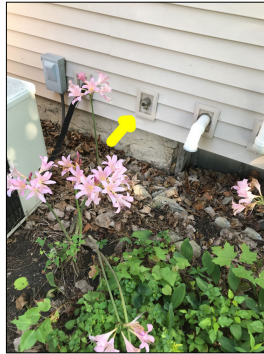
Damaged/missing handle.
