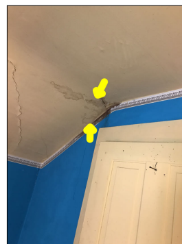
Discoloration along the ceiling and signs of previous water damage. An active or intermittent water source can cause mold growth and property damage.
