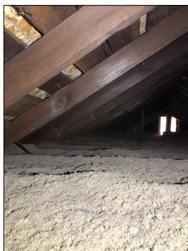
General photo of the attic.
