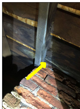
Signs of previous water damage along the sheathing. An active or intermittent water source can cause mold growth and property damage, such as wood rot damage.
