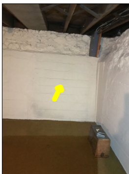
Structural modifications and repairs observed along the foundation walls.
