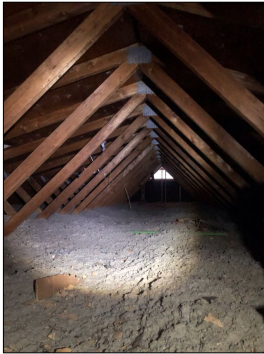
General photo of the attic.
