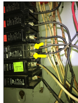
Rust and corrosion within the circuit breaker panel. This is considered abnormal and a potential safety hazard. An active or intermittent water source can cause rust and corrosion. Rusted/corroded terminals and connections increase resistance in the circuit that can cause overheating, thus causing arcing, spark and/or fire. Some areas of rust and corrosion may not be visible and could be concealed behind breakers, wires, etc.
