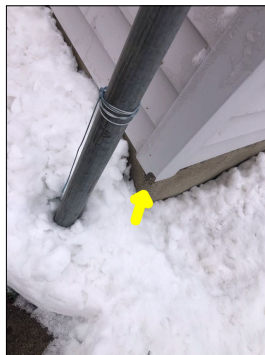
Damaged siding.
