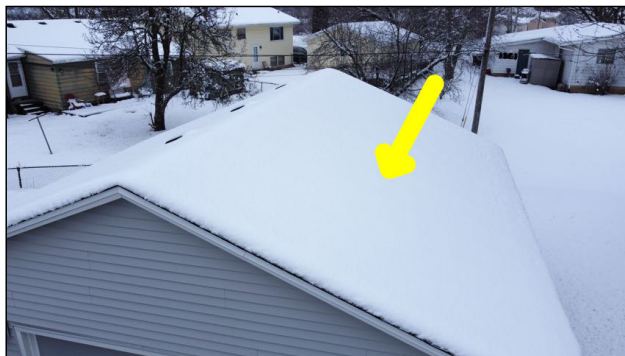
The roof was covered with snow. Visibility and accessibility were limited.
